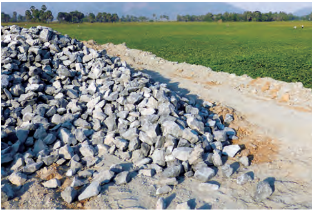
Fig. 5. Granite stone (diameter, about 10 - 15 cm) utilized as roadbed under the asphalt pavement.
